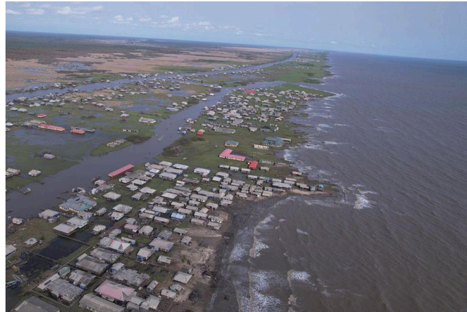
Figure 2: Satellite Imagery of Ayetoro Coastal Community (Source: Oluwatunmise et al, 2025)
