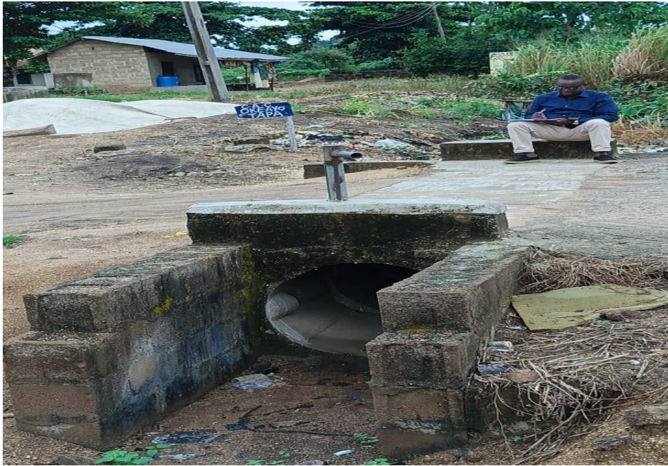
Plate 1: Box culvert constructed by Ayedaade Community Development Association in Tapa (Coordinates: 31N 0524920 UTM 0837405)
