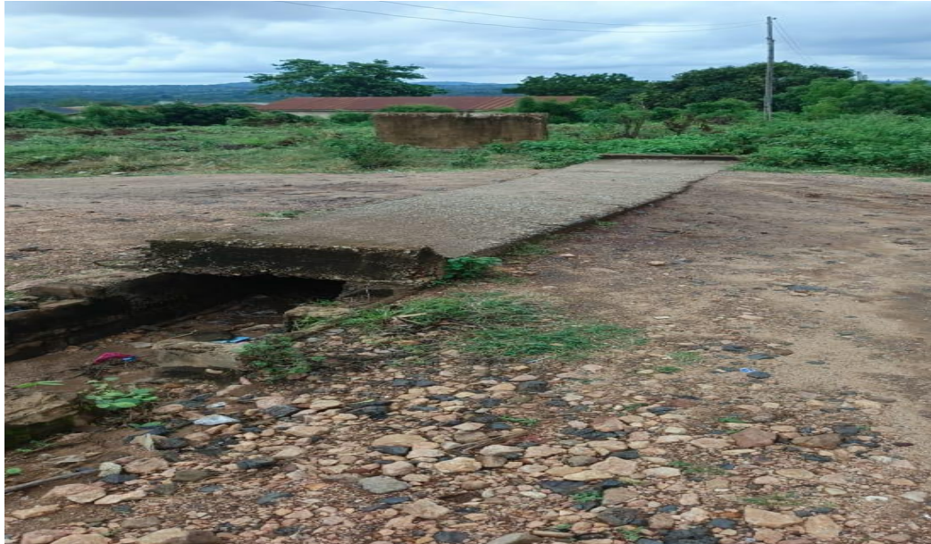
Plate 3: Rehabilitation of Damaged Road Sections through Rubble Filling, Culvert Construction, and Drainage Development by Ifelajulo CDA along Ori Oke Oyinbo–Saganhun Road, Igboora
